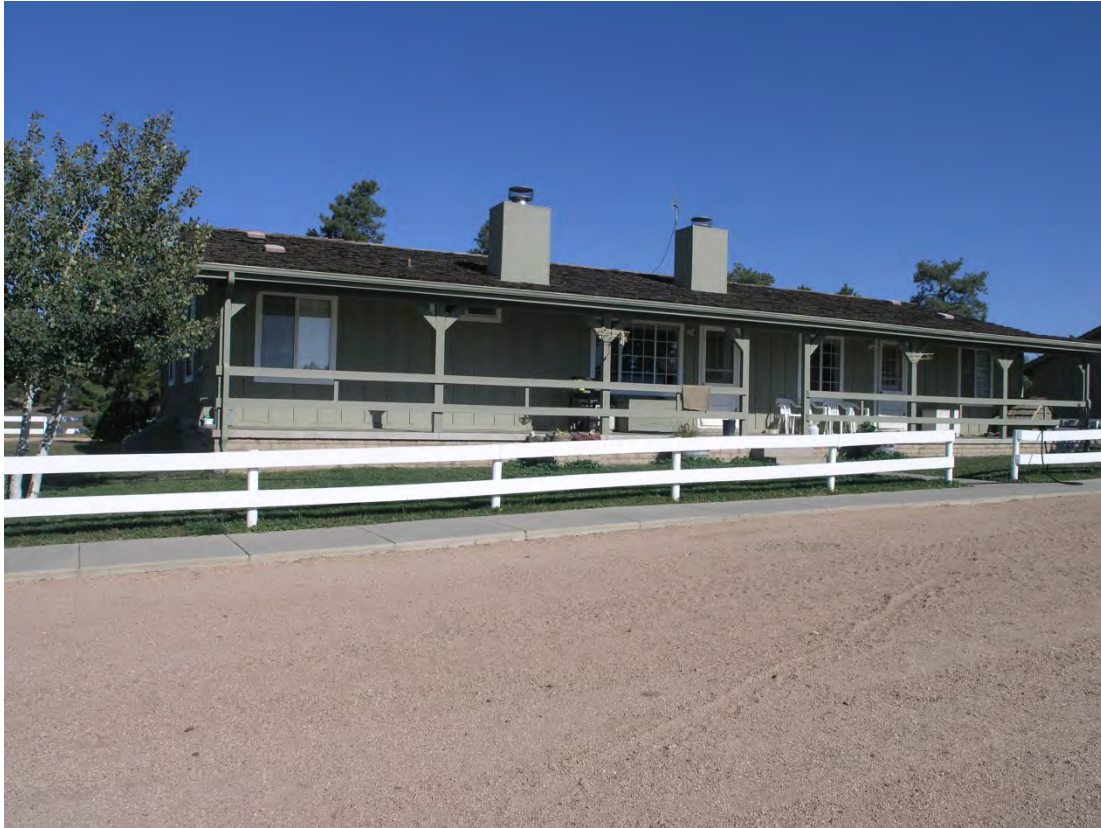
View of the Foreman's residence.
